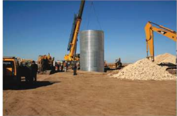
Installation of Outer Can of the foundation
